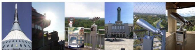
Ještěd tower, Liberec, CZ
